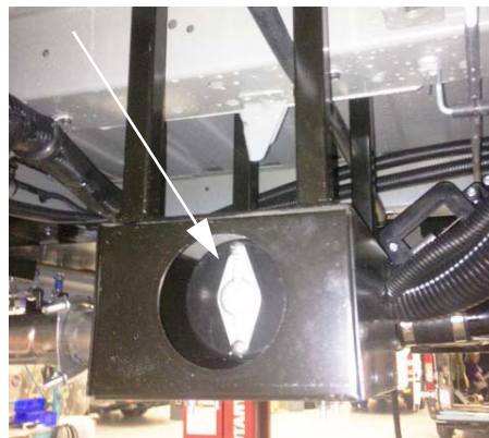
Waste Pump (Located beneath motorhome)
