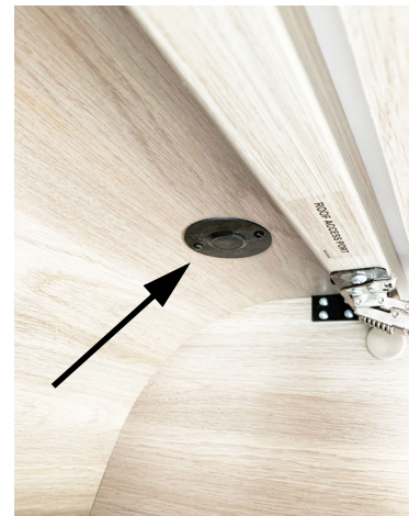
Roof Access Port -Typical View
