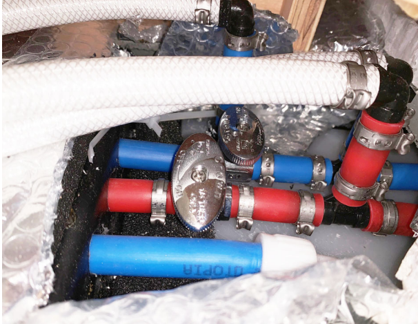
*Model 59G shown (See “Water System Drain Valve Locations” chart at the end of this section for location on your model)
